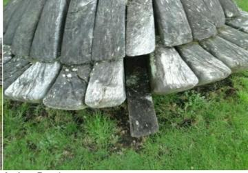
Finding: A timber section has collapsed
