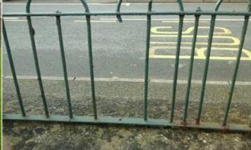
**Finding:** There are a number of poles missing from the **Action:** Replace missing poles
