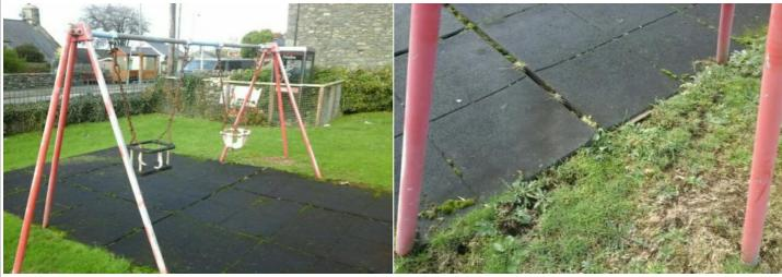
Finding: The tiles can easily be lifted or are lifting along the Action: Lift and re-glue tiles to secure edges of the area
