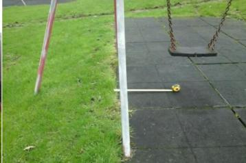
Finding: The seats are too close to the frame as defined in Action: Monitor use BS EN 1176 Part 2; this is a low risk failure and no remedial action is required
