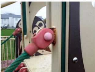
The paintwork on this item has been damaged or worn exposing the metal underneath which is rusting Finding:
