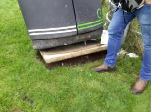
The bin is not securely fixed to the surface and there is some possibility of the item tipping or rolling over Finding:
