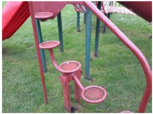
Finding: Rubber bearing worn on seesaw step Action: Replace
