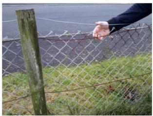
Finding: There are projecting wires Action: repair
