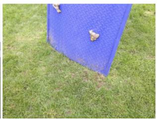
Finding: Climbing wall loose in ground at base Action: Re concrete
