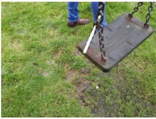
**Finding:** The chain openings are in excess of the 8.6mm as recommended by BS EN 1176
