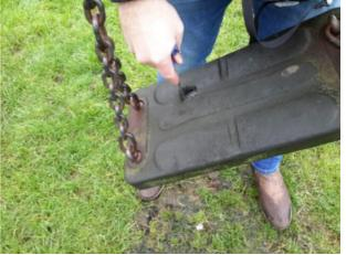
**Finding:** The seat is severely damaged and requires
