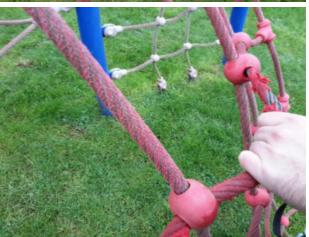
**Finding:** The ropes/nets are worn/damaged in places
