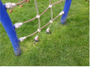
**Finding:** The grass mats are silted up and the soil is compacted; this may have an effect on the impact absorbing properties of the surface
