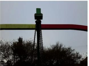
Finding: Swings of this design should have a secondary safety mechanism fitted unless the joint has been designed and tested
