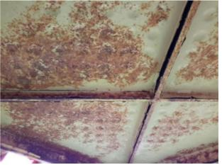
Finding: The paintwork on this item has been damaged or worn exposing the metal underneath which is rusting under the
