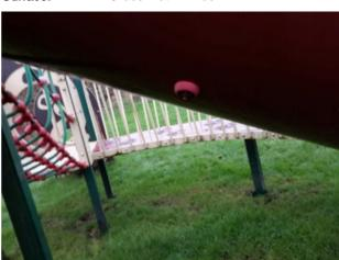
There is/are bolt cap covers missing or damaged on the item Finding:
