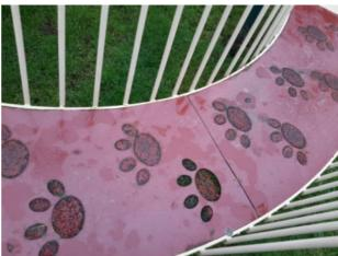
Finding: Wetpour inlays are worn Action: Repair
