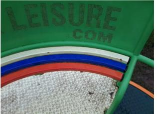
Finding: The paintwork on this item has been damaged or worn exposing the metal
