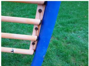
Finding: Fixings have corroded Action: Replace
