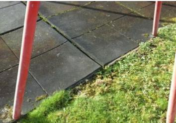
Finding: The tiles can easily be lifted or are lifting along the Action: Lift and re-glue tiles to secure edges of the area
