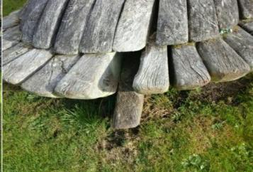
**Finding:** A timber section has dropped allowing a foot entrapment
