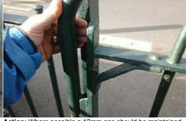
**Finding:** The opening between the gate and the post or the double gate leafs is less than 12mm and could trap users
