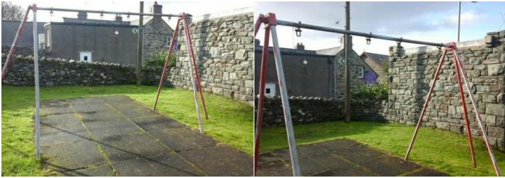
**Finding:** The seat(s) and suspension were missing at the time of inspection and the inspector was unable to make a full compliance assessment
