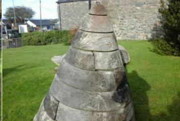
Finding: The top section is loose Action: Secure top section
