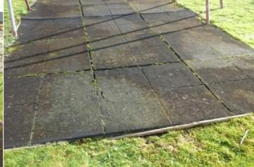
Finding: There are trip hazards at the edges of the surface Action: Reinstate surrounding surface levels to remove the trip points
