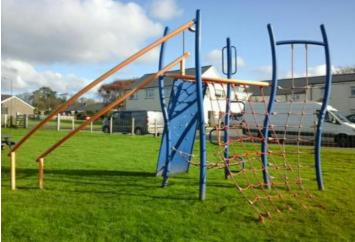
Finding: The climb wall is slightly loose in its foundations
