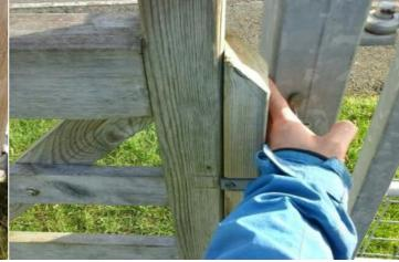
Finding: The opening between the gate and the post or the Action: Where possible a 12mm gap should be maintained double gate leafs is less than 12mm and could trap users fingers
