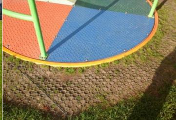
Finding: There are trip hazards present on the roundabout Action: Reinstate surrounding surfaces to level to remove the trip points
