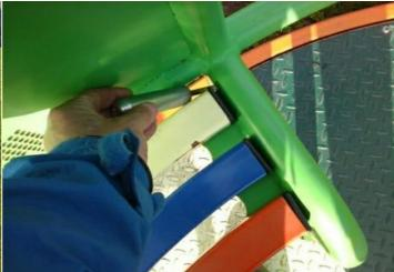
**Finding:** There is/are finger entrapment/s in the framework and the item fails to meet the requirements of BS EN 1176 **Action:** Monitor - No remedial work recommended and the item fails to meet the requirements of BS EN 1176 Part 1 4.2.7.6 Entrapment of fingers
