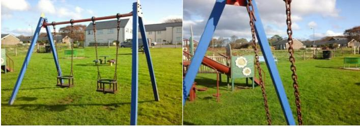
Finding: Chains have corroded Action: Monitor and replace as required
