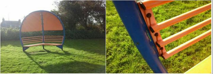
Finding: Fixings have corroded Action: Replace
