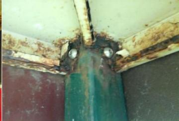
**Finding:** There is heavy corrosion to the platforms fixing points
